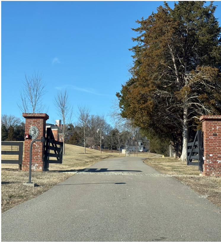
Gates at entrance
