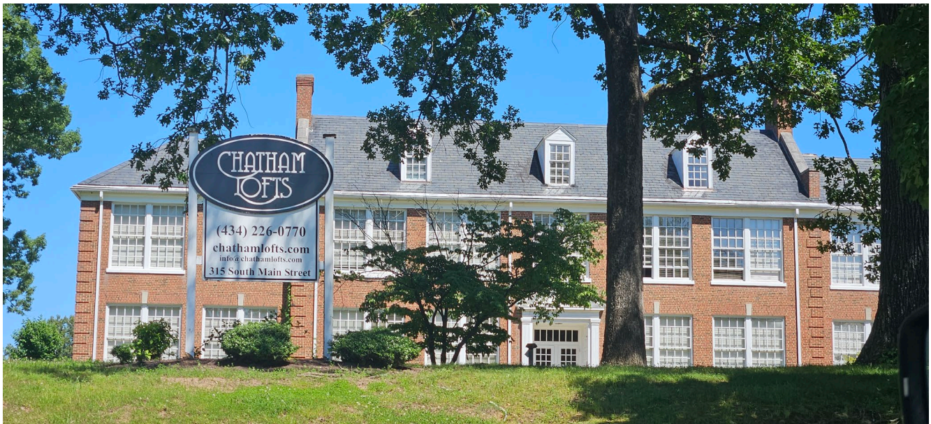
Chatham Lofts, a 31-unit apartment building that was a renovation of a 1920's school.
